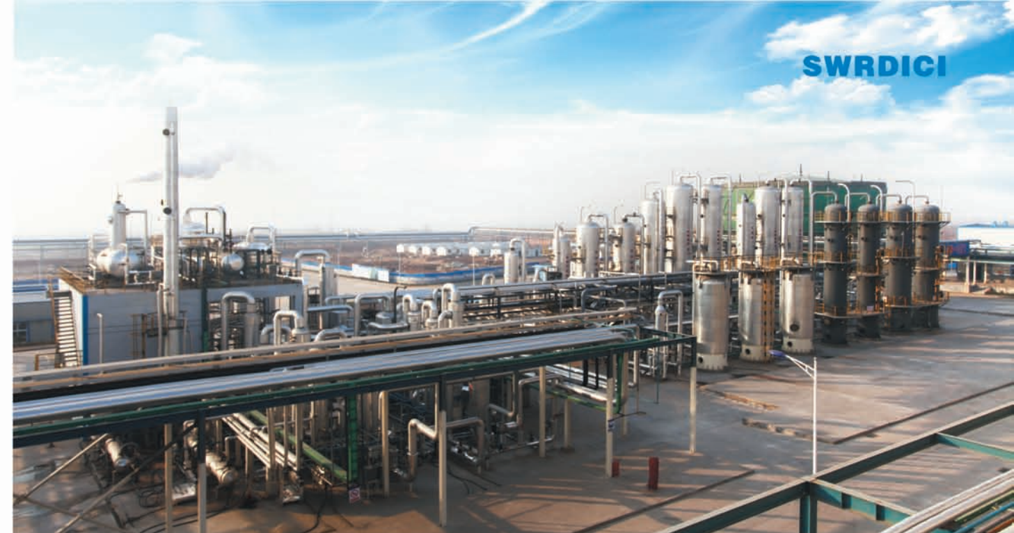
河北裕泰集团有限公司（30000Nm 3 /h）焦炉气制压缩天然气(CNG)工业装置 Plant for producing compressed natural gas (CNG) from 30000Nm 3 /h coke oven gas in Hebei Yutai Group Co., Ltd
