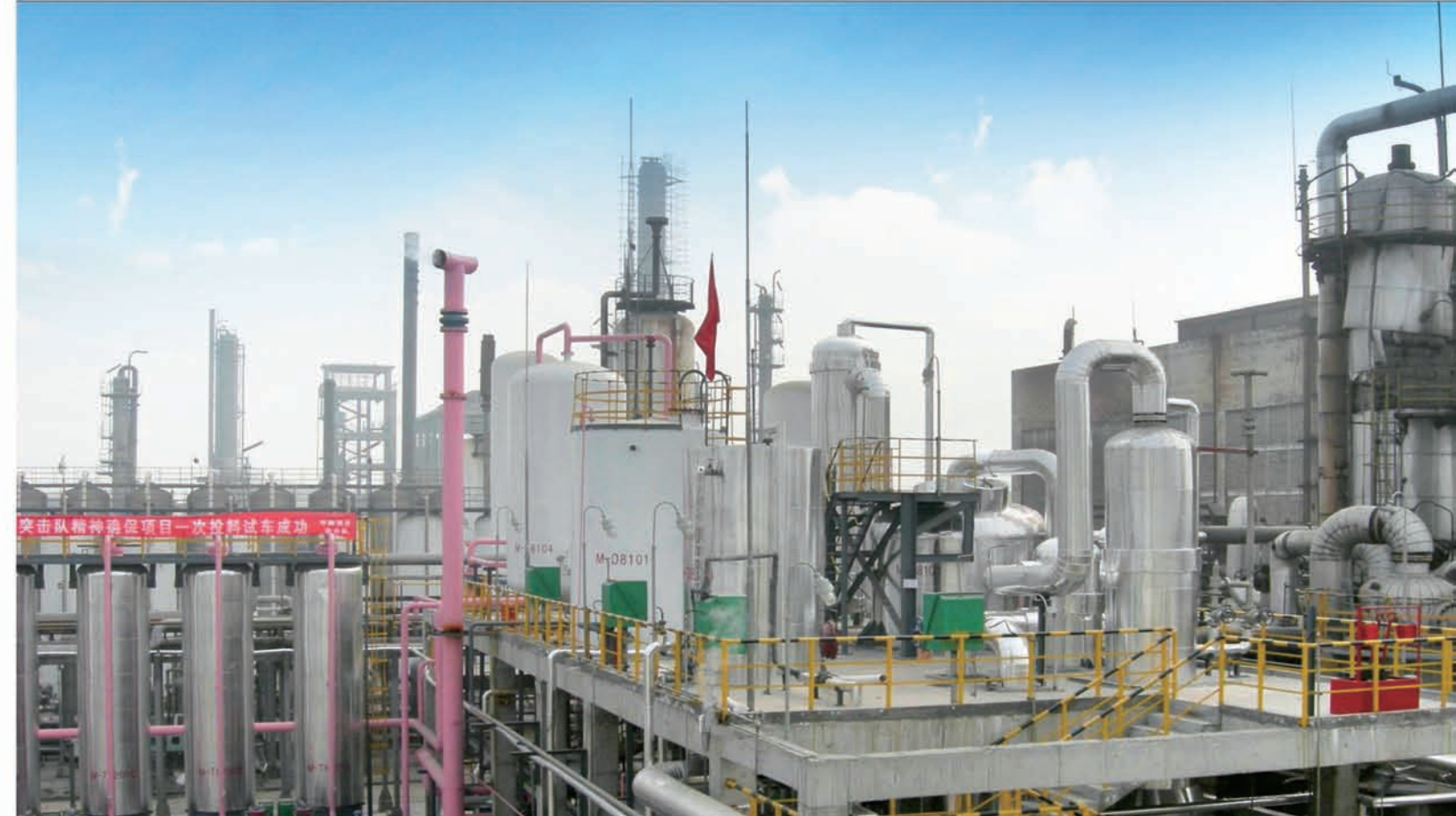
河南神马尼龙公司4000m³/h甲醇制氢工业装置 4000m³/h methanol-to-hydrogen plant in Henan Shenma Nylon Chemical Co., Ltd.
