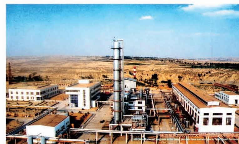
榆林天然气化工厂甲醇工业装置（首套国产化万吨级装置） Methanol plant in YUTIAN HUA - first natural gas-based methanol facility in China with the capacity of more than 10 thousand tons annually
