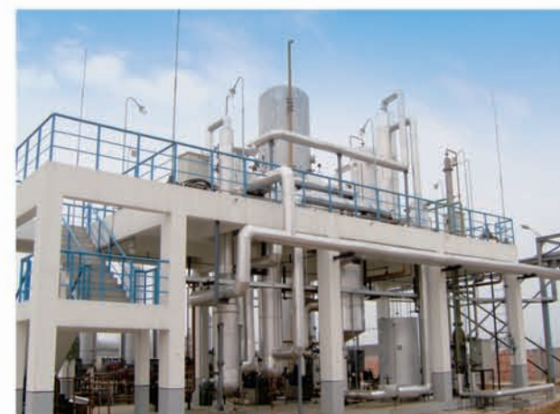
东北制药厂1000Nm³/h甲醇制氢装置 1000m³/h methanol-to-hydrogen plant in Dongbei Pharmaceutical Factory
