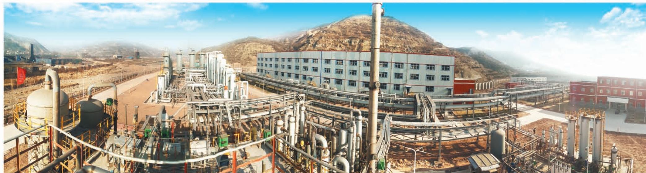
山西国新正泰新能源有限公司（30000Nm 3 /h）焦炉气制合成天然气(SNG)工业装置 Plant for producing synthetic natural gas (SNG) from 30000Nm 3 /h coke oven gas in Guoxin Zhengtai New Energy Source Co., Ltd.
