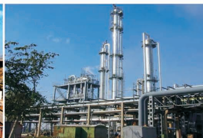
锦西天然气化工公司3万吨/年合成氨联产甲醇装置 30kt/a methanol plant combining with ammonia synthesis system in Jinxi Natural Gas Chemical Co., Ltd.
