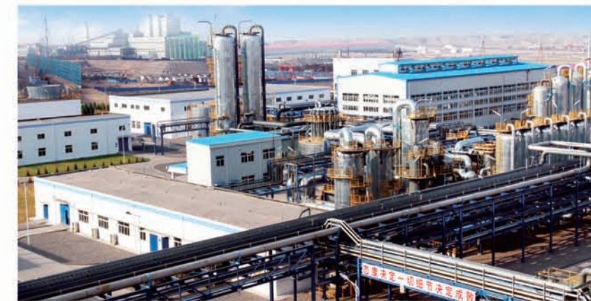
河北裕泰集团有限公司（30000Nm 3 /h）焦炉气制压缩天然气(CNG)工业装置 Plant for producing compressed natural gas (CNG) from 30000Nm 3 /h coke oven gas in Hebei Yutai Group Co., Ltd
